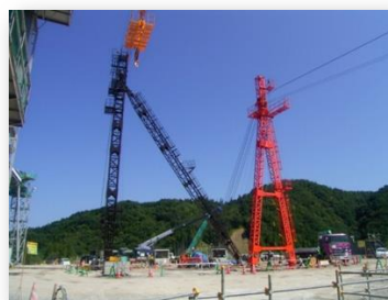
Cable Cranes for Dam Construction
