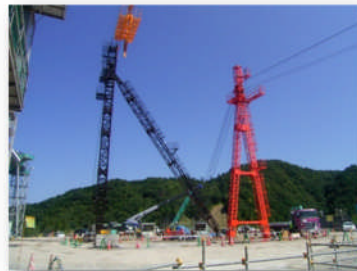
Cable Cranes for Dam Construction
